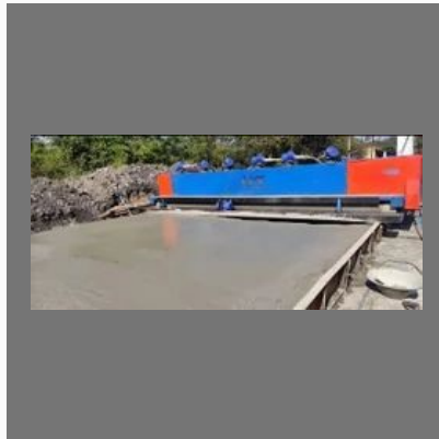
Vibrating Road Paver
